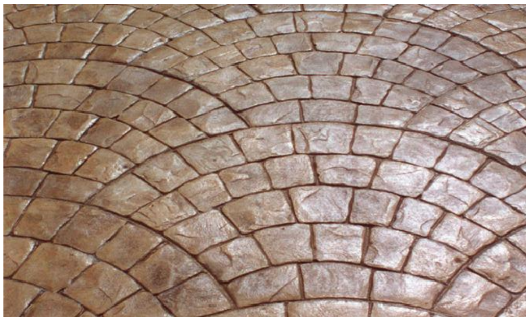
STAMPED CONCRETE EXAMPLES
